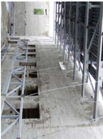
Construction of Elevated Running Track
