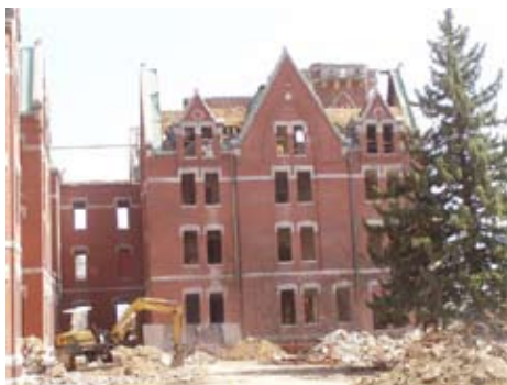
Kirkbride Building "Under Rehab"
