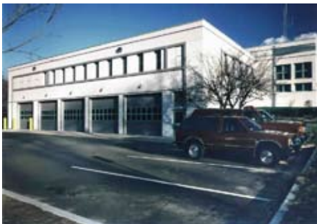
Ludlow Police & Fire Ludlow, Massachusetts
