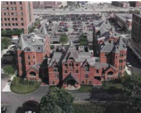
Boston University's Talbot Building Boston, Massachusetts Photo by Peter Vanderwarker
