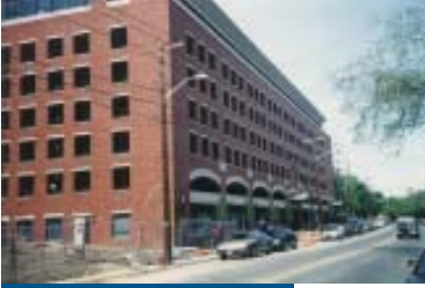
Tufts University Parking Garage Medford, Massachusetts Architect: ADD, Inc.
